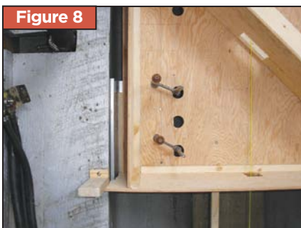
Figure 8 Marking the stringers for the new brackets.
