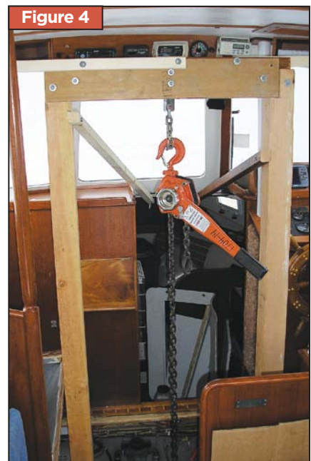
Engine hoisting arrangement.
