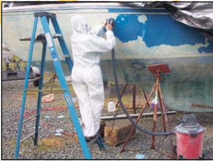
Proper set up for sanding: eye protection, respirator, bunny suit and a shop vac for dust.
