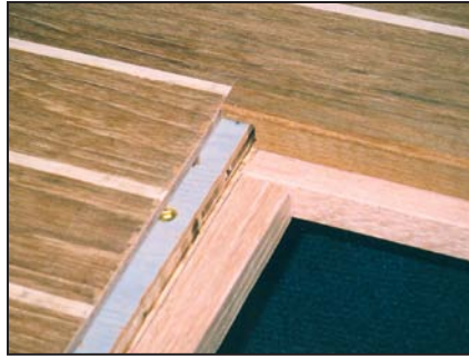
Hatch opening detail with back molding in place. Note corner detail.
