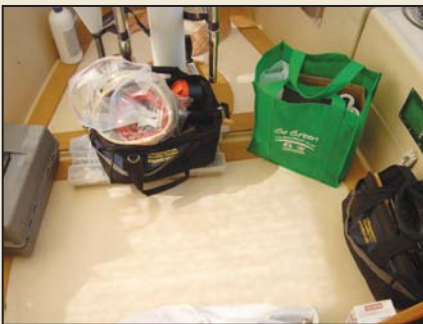
Bedded perimeter planks weighted down for an overnight cure.
