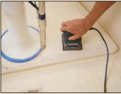
Sanding the fiberglass cockpit floor.
