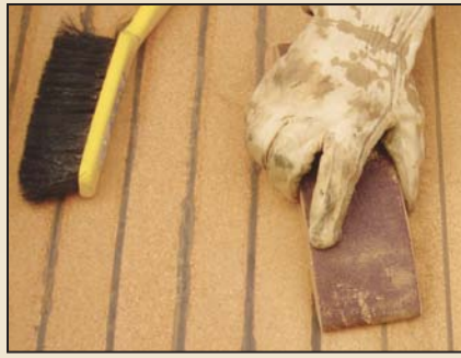
Hand sanding excess cured caulking compound. Note before and after sanding!
