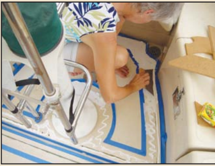
Applying white bedding compound.
