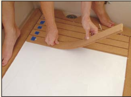
Rolling planks into position over the bedding compound.
