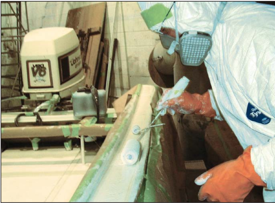
Rolling on a polyurethane stucco non-skid.
