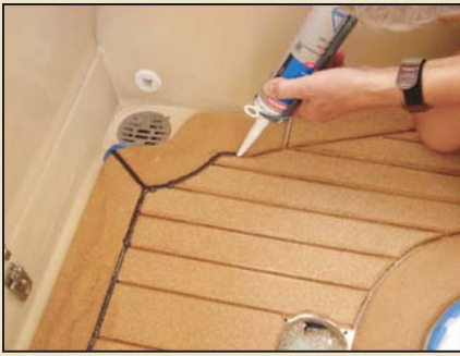
Applying black seam caulking compound.
