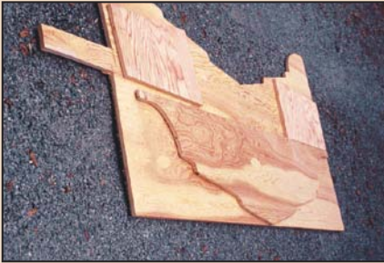
Marine-grade plywood is cut into sections to facilitate installation.
