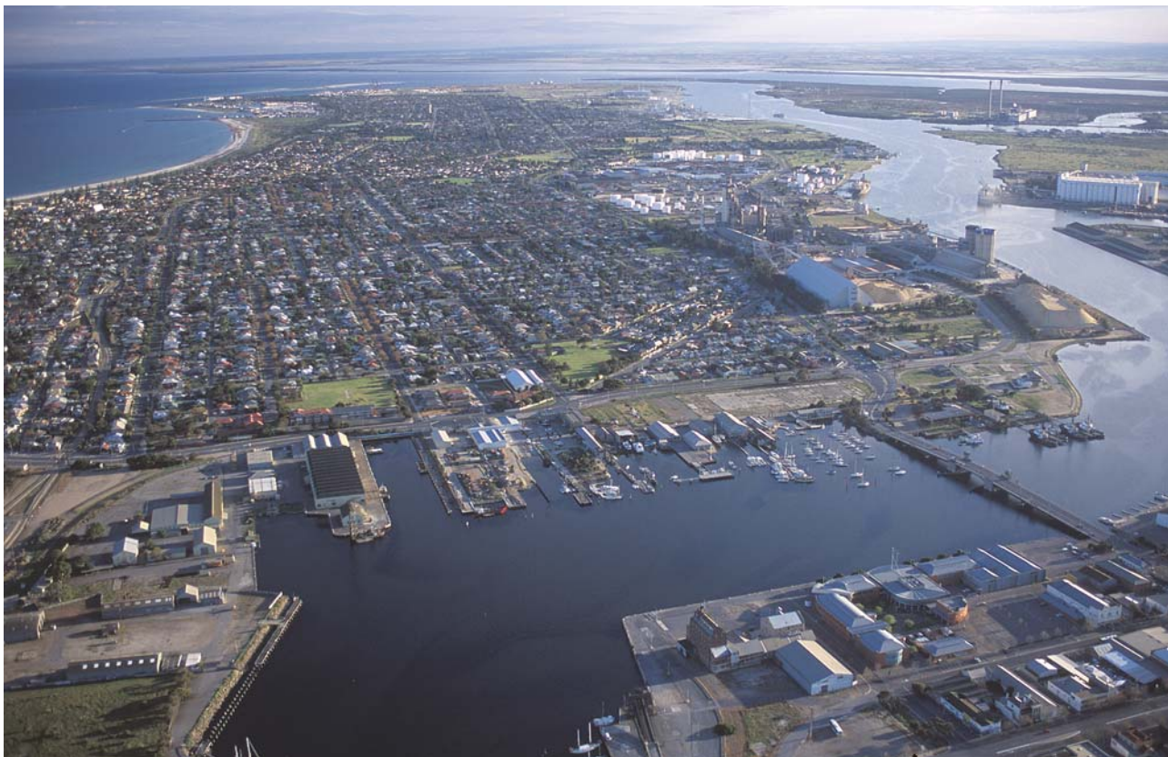
Port Adelaide – Birkenhead Bridge (12.140)
