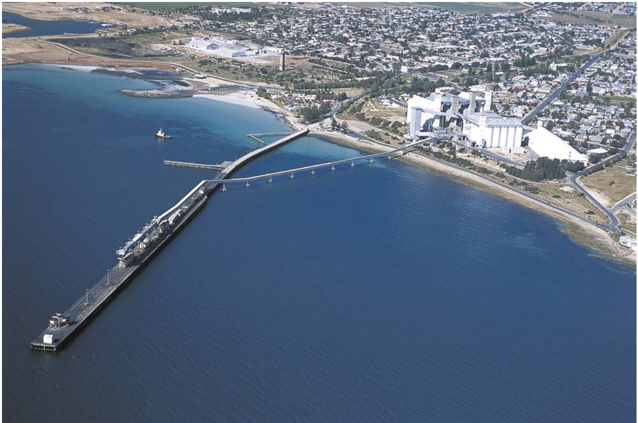
Wallaroo Jetty and Silos (11.125)
