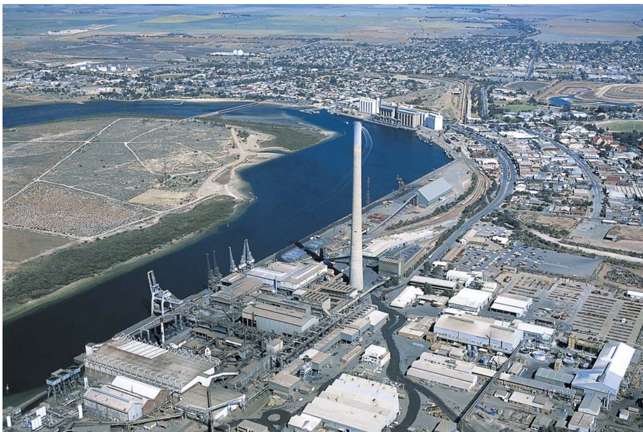
Chimney at Pirie Port (11.200)
