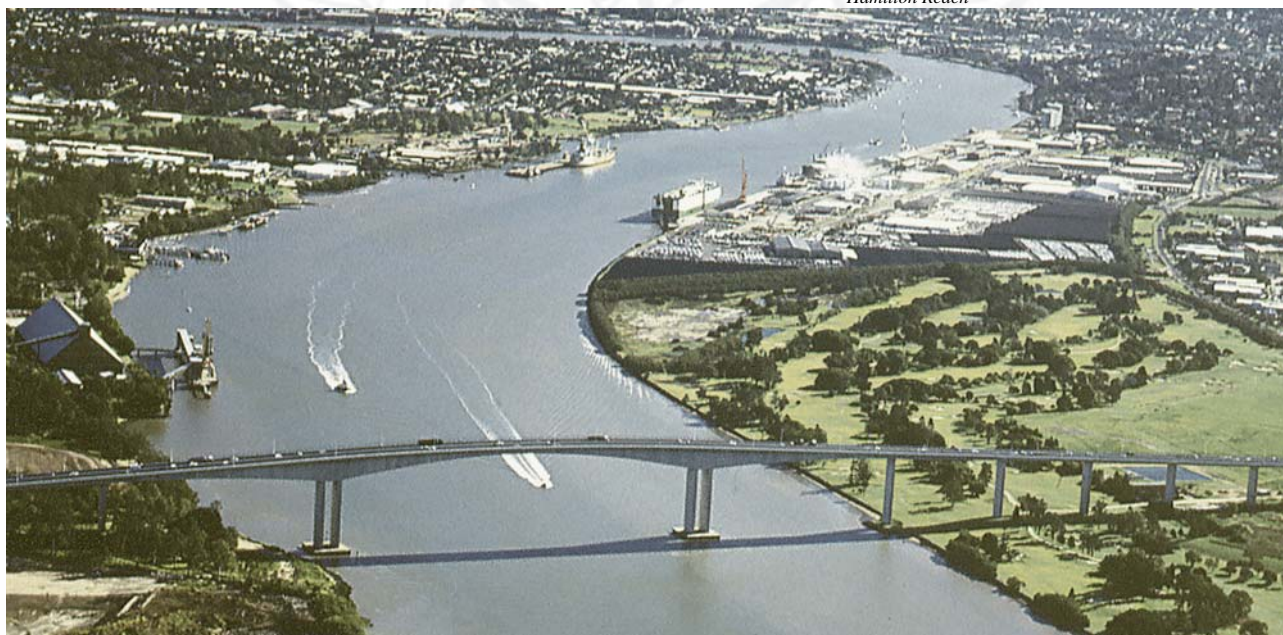
Gateway Bridge from NE (4.86) (Original dated 1999)
