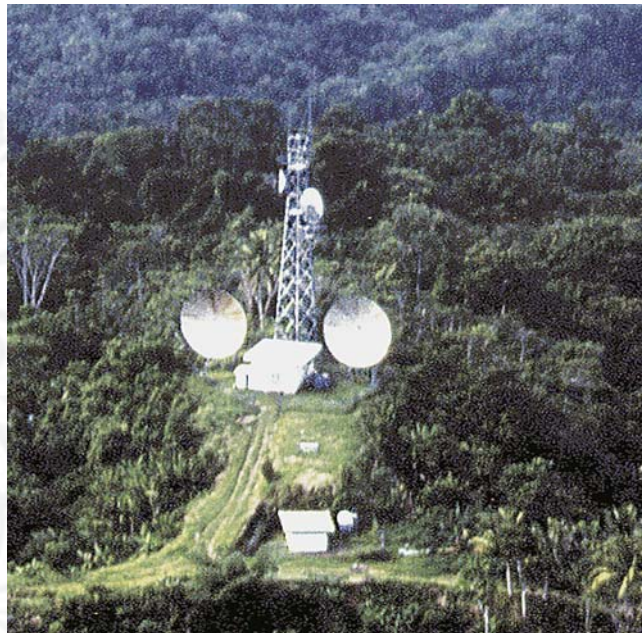
Cape Cupola radio tower (12.186)
