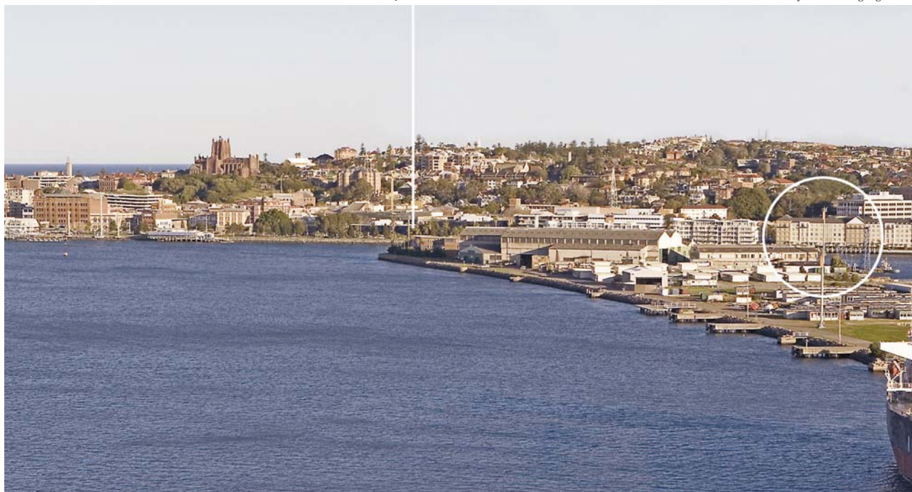
Steelworks Channel from N (3.117)
