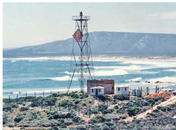
Quoin Point Light (10.147)
