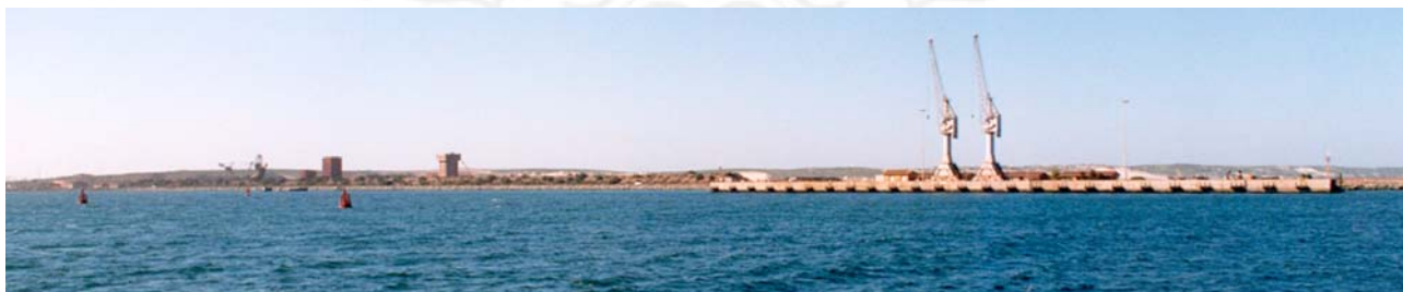
Saldanha Bay Harbour – Multi Purpose Terminal (9.151)
