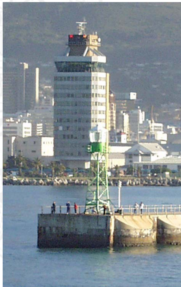
Cape Town Port Control building (9.235)
