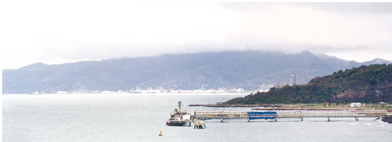
Asahimas Chemical Jetty from SW (2.52)
