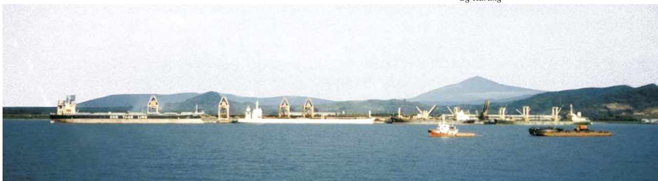
Cigading Ore Jetty berths (2.60)
