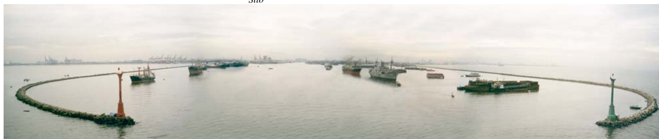
East breakwater light-structure
