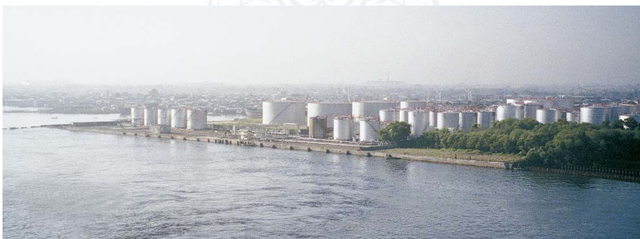
Tanjungpriok DKP Chemicals Berth from WNW (3.166)
