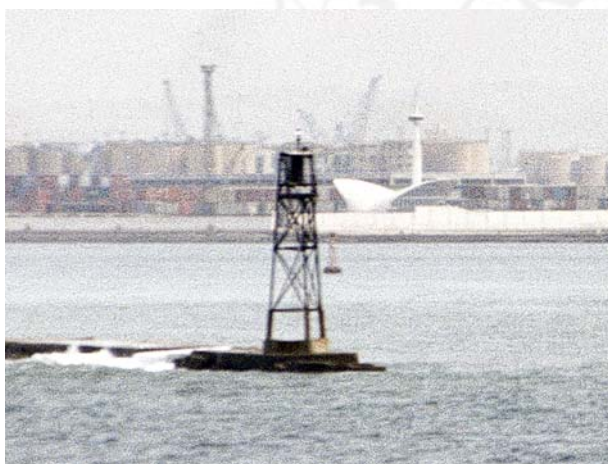
Manora Point Breakwater Light from S (10.121)
