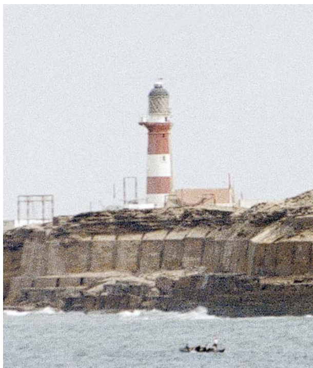
Manora Point Lighthouse from NE (10.118)
