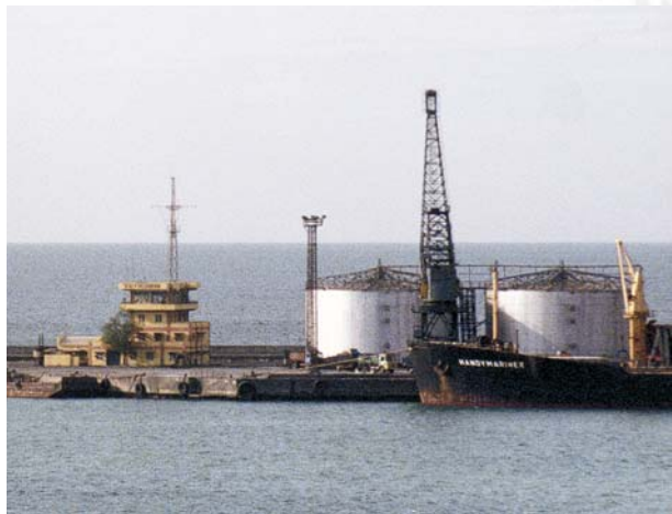
Signal Station E Breakwater from N (4.184)
