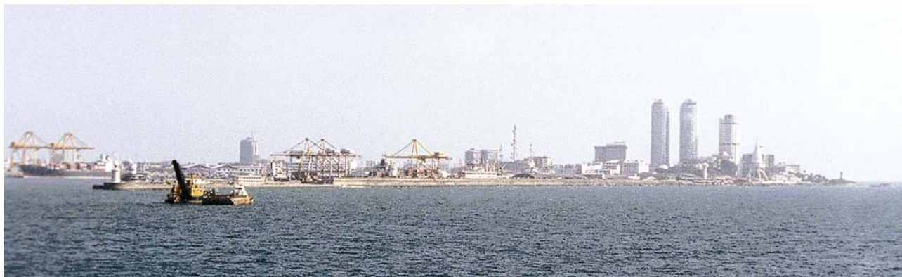
SW Breakwater Head
