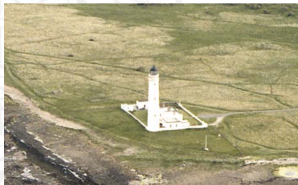
Barns Ness Lighthouse from NE (5.13.2)
