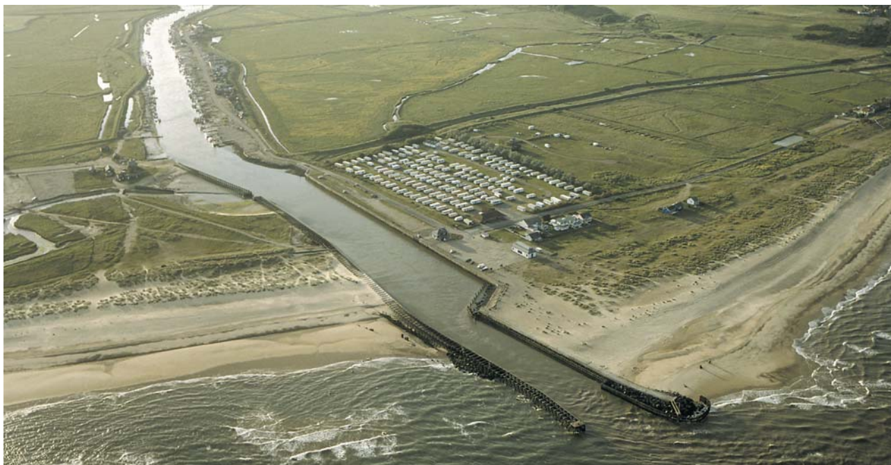
Southwold Harbour from S (9.135) (Original dated 2000)
