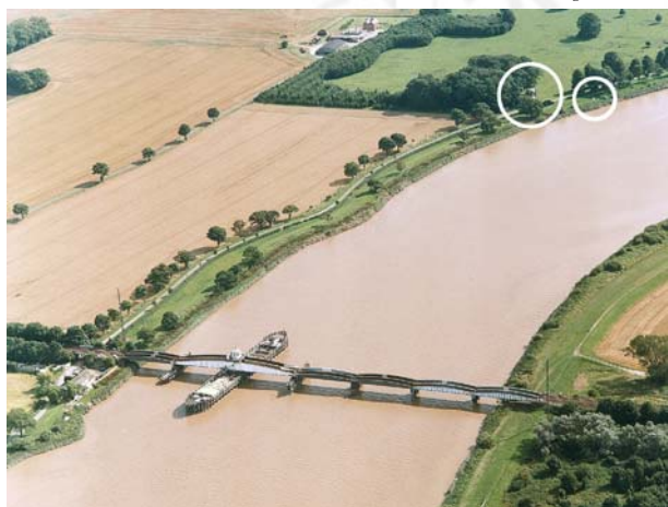
Skelton Railway Bridge from N (7.153)
