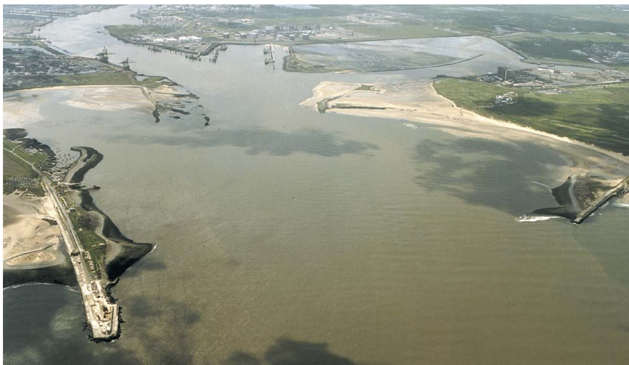
South Gare Breakwater
