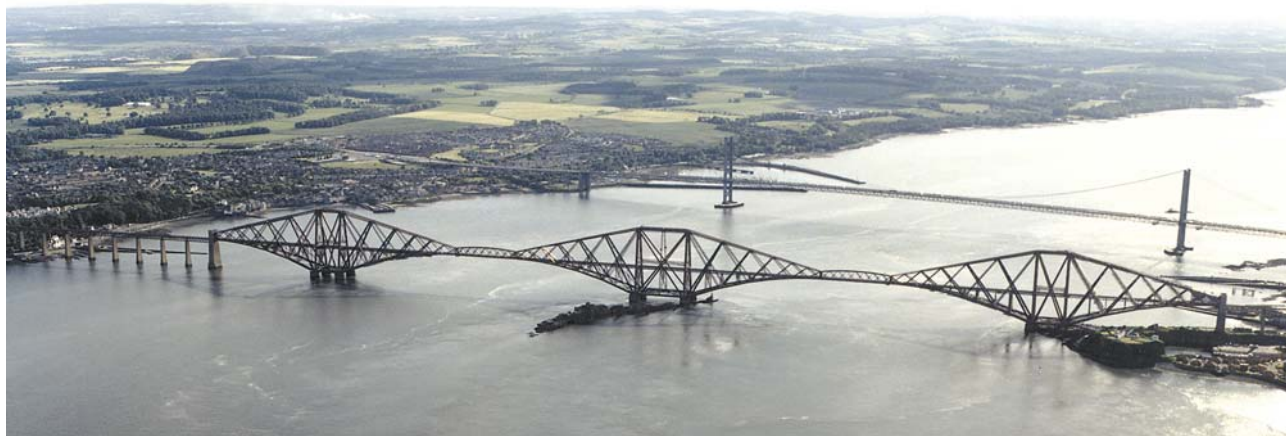
Forth bridges from NE (4.133.1)
