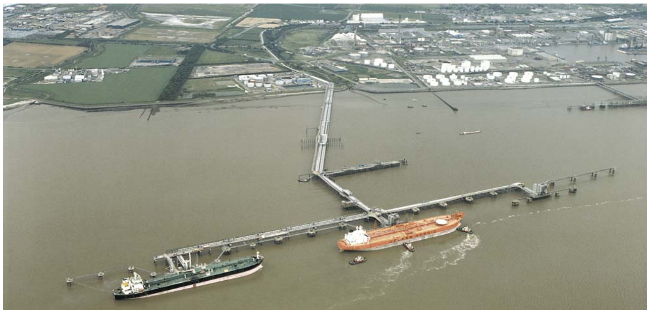
Immingham Oil Terminal from NE (7.87)
