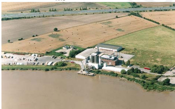
Howdendyke W Jetty from S (7.174.1)
