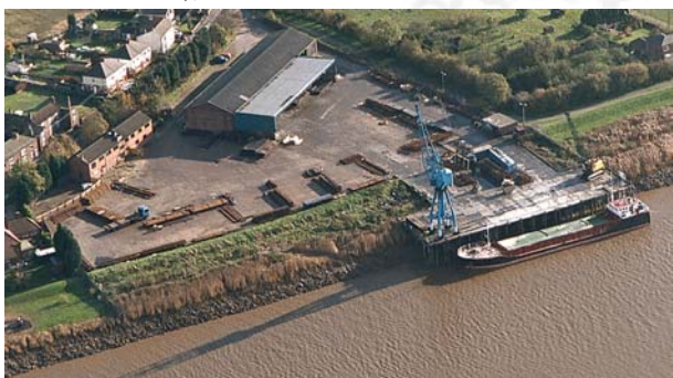
King's Ferry Wharf from NW (7.179)
