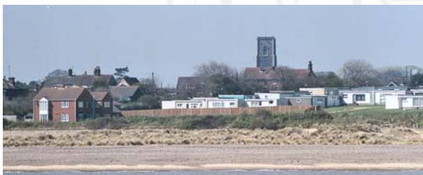
Kessingland Church (tower) from E (9.132) (Original dated 2002)
