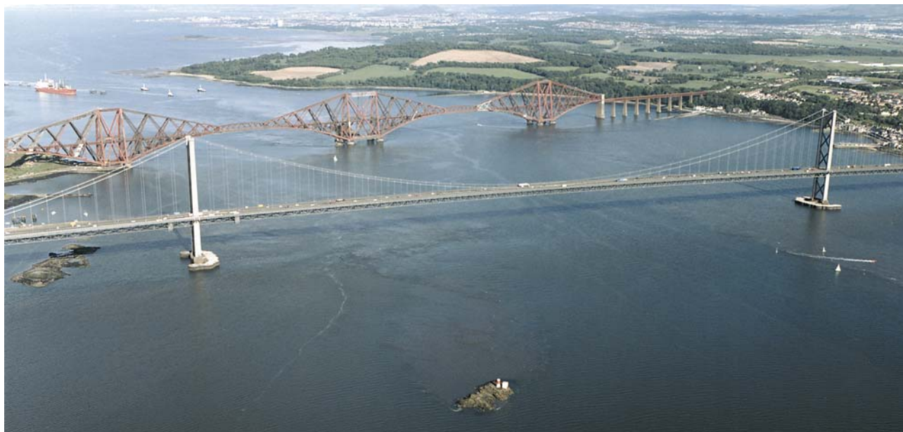
Beamer Rock Forth bridges from NW (4.133.2) (Original dated 2000)
