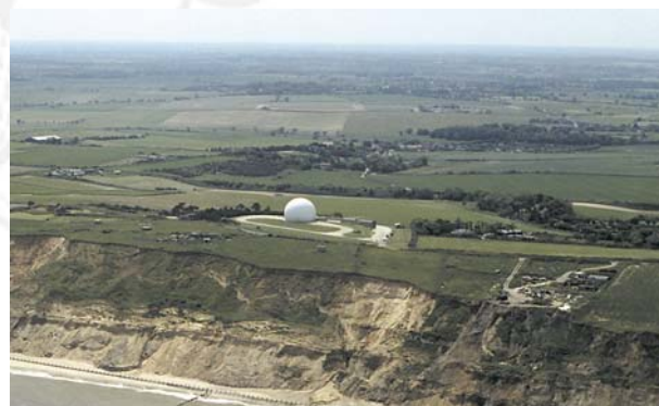
Radome at Trimmingham from NNE (9.22)
