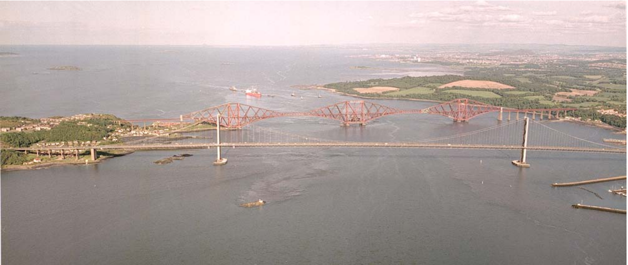
Forth Bridges from W (4.133) (Original dated 2000)
