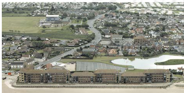
Conspicuous building, Mablethorpe from ENE (8.12)
