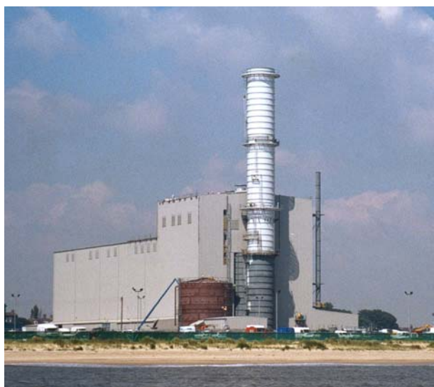
South Denes Power Station from ESE (9.47)
