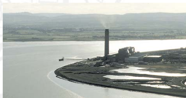
Longannet Power Station chimney from E (4.224)
