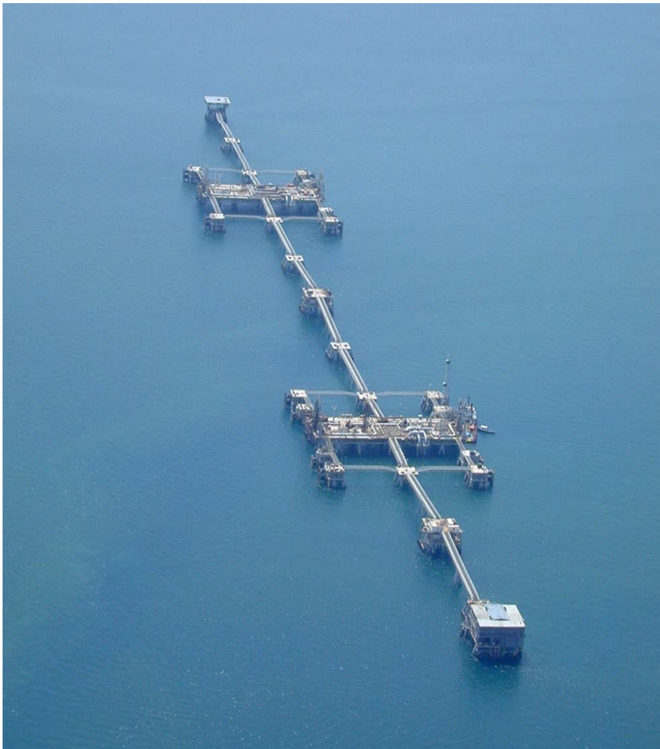
Al Basrah (Al Bakr) Oil Terminal W (9.90)
