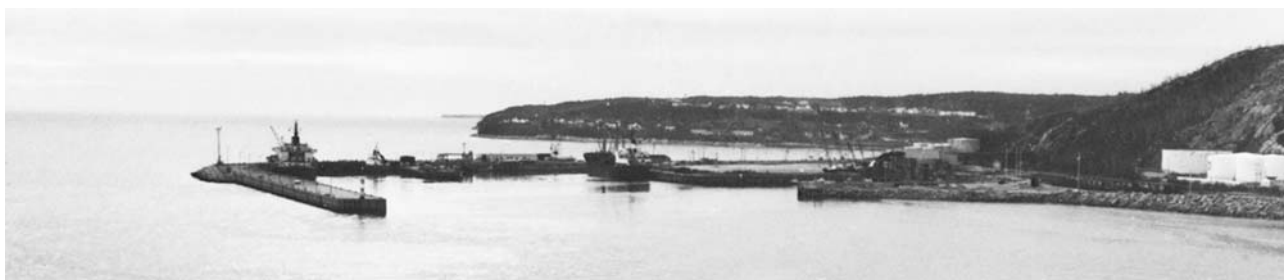
Baie-Comeau Dock No 1 (5.179)
