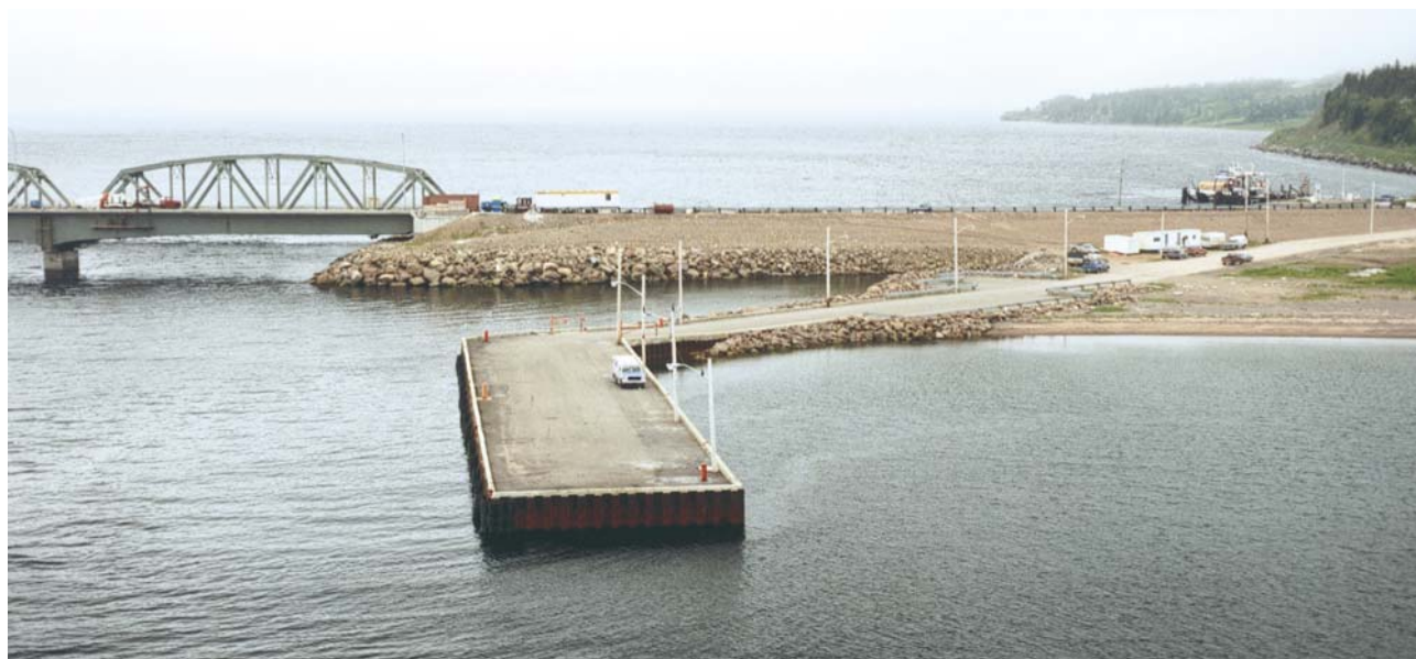
Cape Breton Island, Iona Wharf (11.162)
