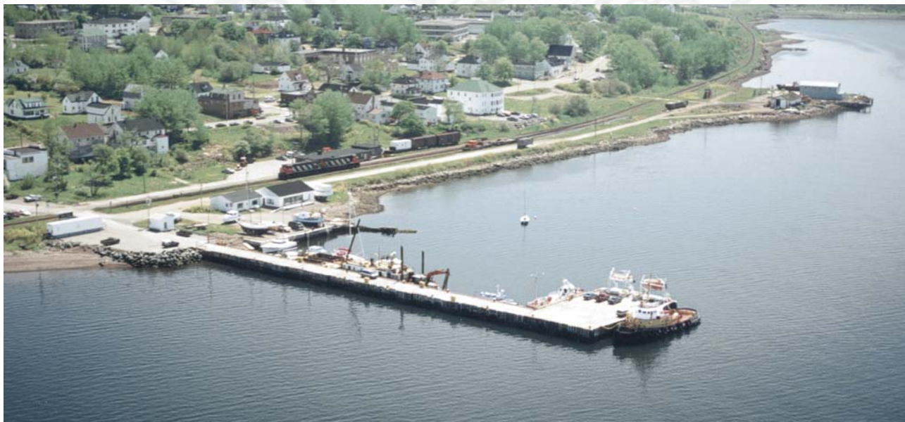
Port Hawkesbury Wharf (12.207)
