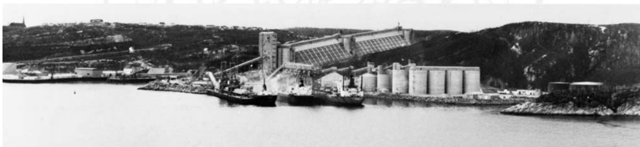
Baie-Comeau Dock No 3 – Cargill Grain Terminal (5.179)
