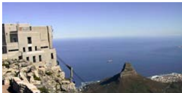
Upper Cable Station (Table Mountain)
