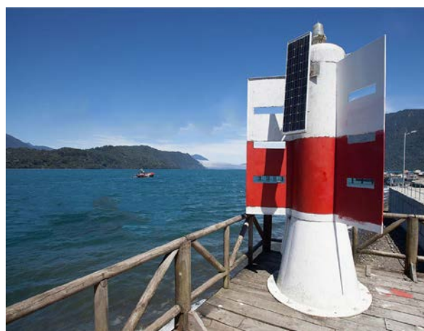
Calbuco Pier Light
