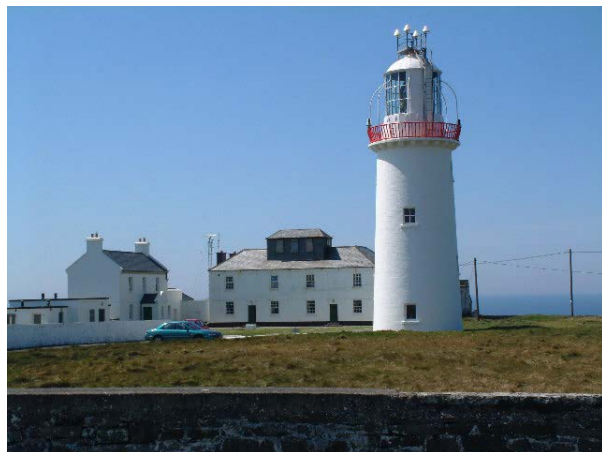
Courtesy of the Commissioners of Irish Lights Loop Head Light
