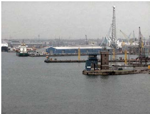
Courtesy of USCGC CAMPBELL Dublin—Port Radio/Radar Station
