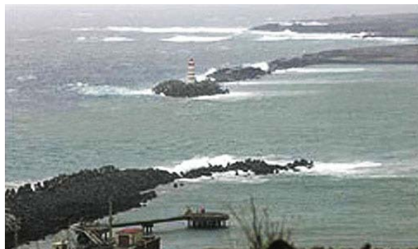
Terceira Light and breakwater
