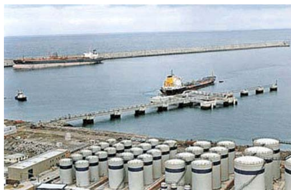
Bilbao—Punta Lucera Breakwater from SE
