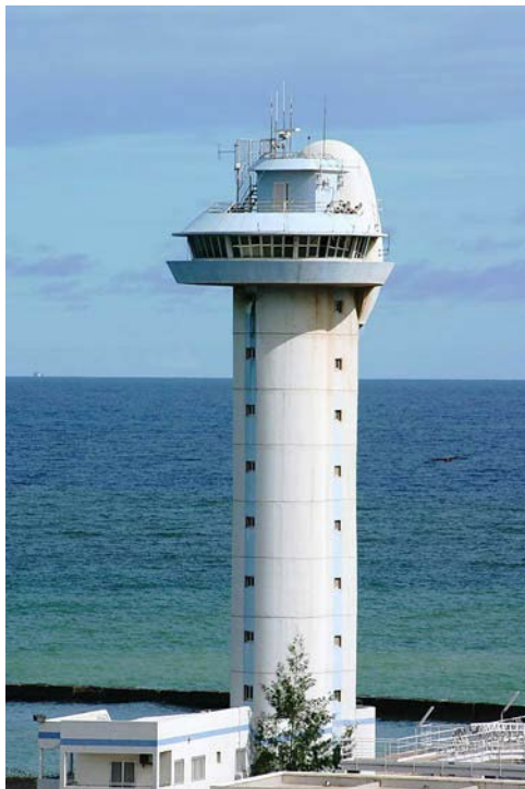
Dakar Harbor Control Tower
