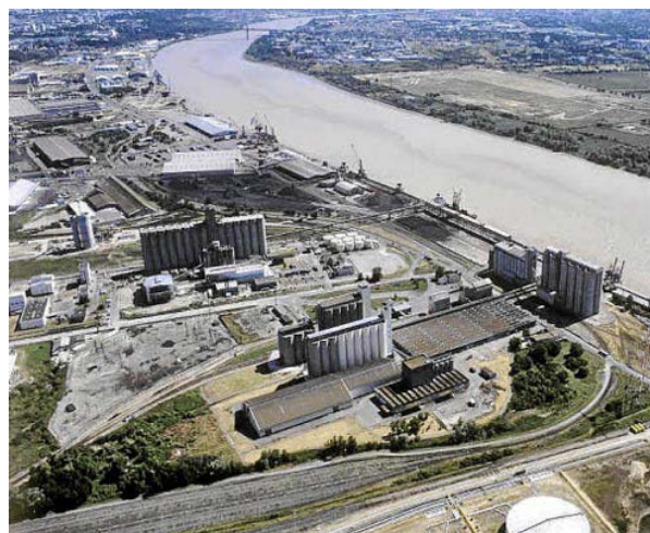
Bordeaux—Dry Bulk and Timber Quay
