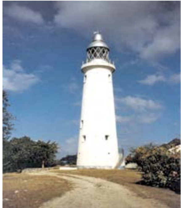
South Negril Point Light
