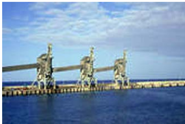
Bridgetown—Conspicuous Sugar-loading Towers
