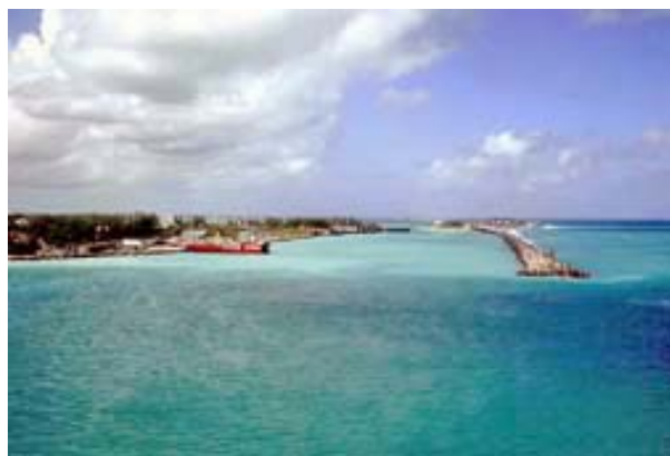
Arawak Cay—West Breakwater
