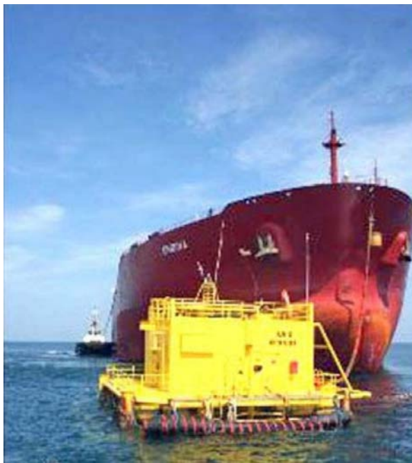
Covenas Tanker Loading Unit (TLU-2)
