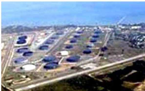
Covenas Tank Farm
