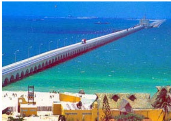
Progreso—Terminal Remota Pier
