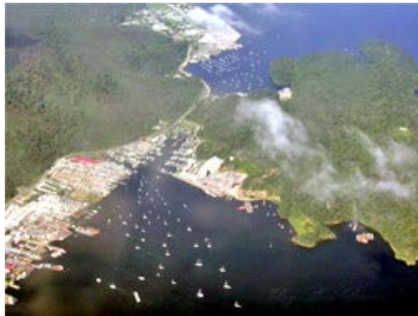
Chaguaramas Terminal Wharf (center)
