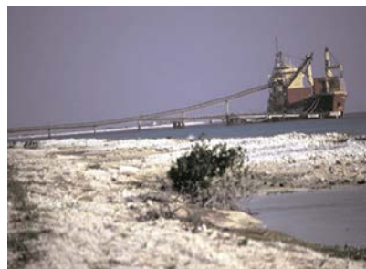
Zoutsteiger Pier (for bulk salt)
