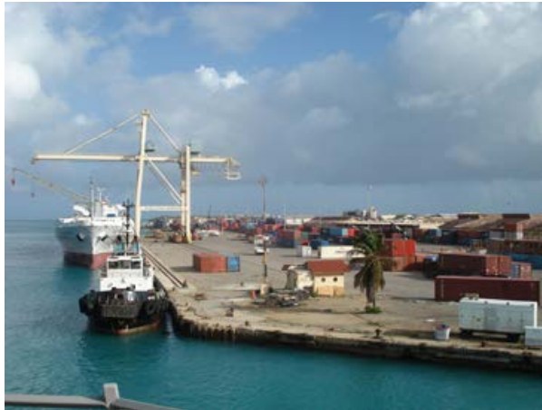
Parden Baai—Container Terminal
