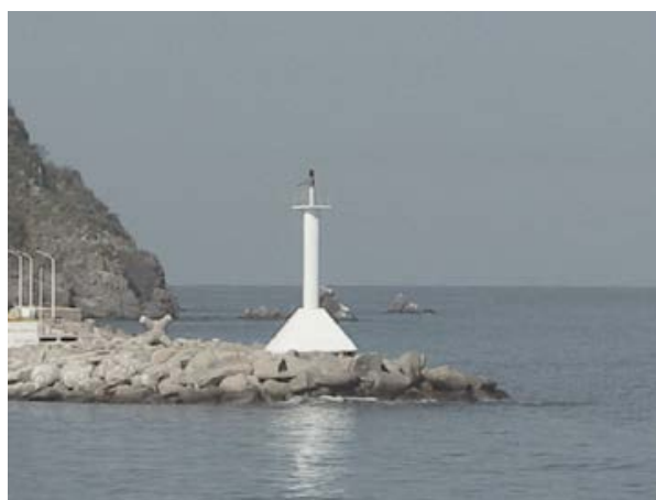
Manzanillo—Northwest Breakwater Light
