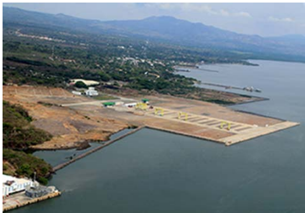
Puerto La Union Wharf from SE
