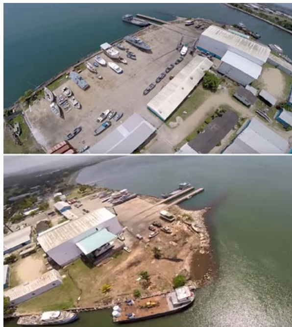
Puerto Cortes Naval Port Piers W of Isla Santa Margarita
