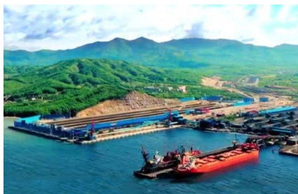
Vostochnyy Coal Handling Terminal
