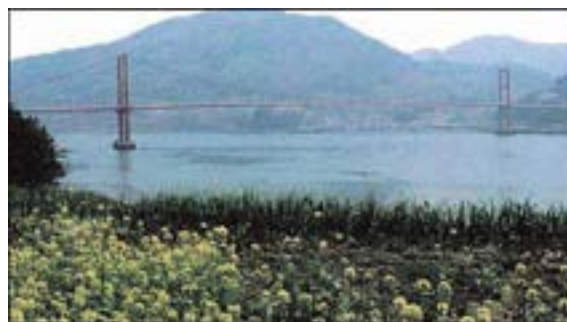
The Tolsan Bridge
