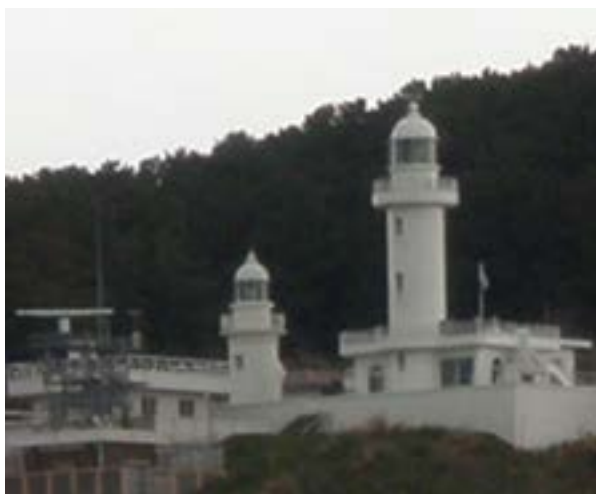
Cheju Hang Traffic Control Center
