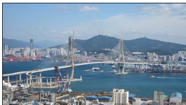
The Bukhang Bridge
