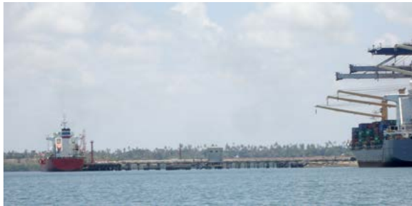
Dar es Salaam Harbor—Kurasini Oil Jetty
