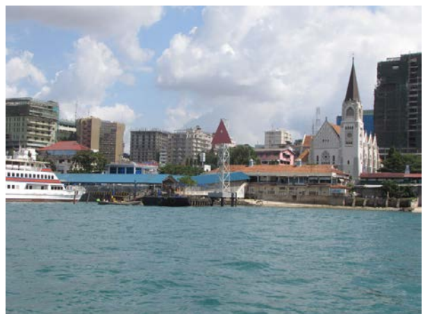
Dar es Salaam Harbor—Passenger Pontoon Pier
