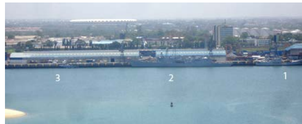
Dar es Salaam—Berths 1 through 3
