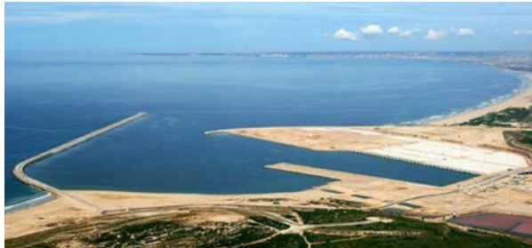
Port Ngqura—Aerial view
