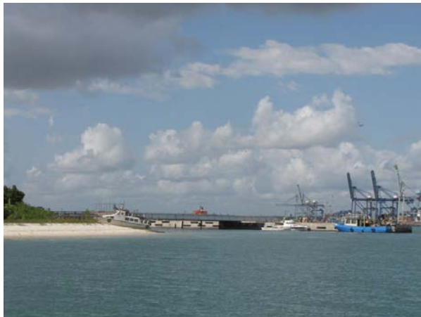
Dar es Salaam Harbor—Tafico Jetty
