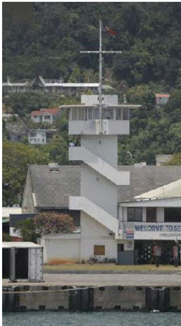
Port Victoria Control Tower/Signal Station
