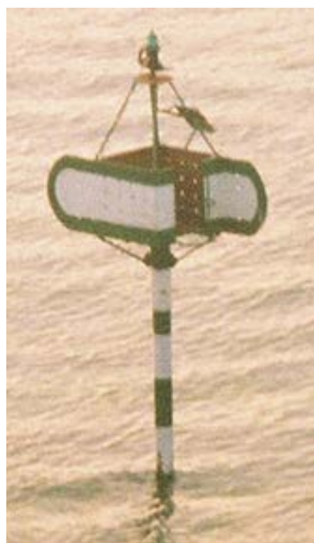
Suez Canal—Typical E side channel marker
