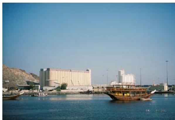
Mina Qabus—Grain Silos
