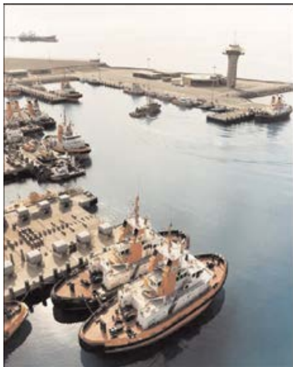
King Fahd Port Control Tower
