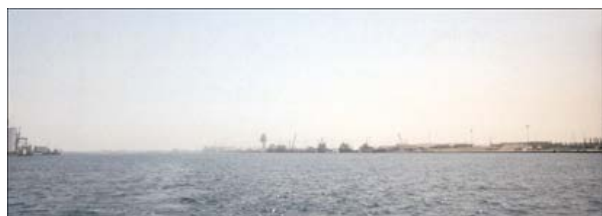
Mina Jabal Ali—Entrance approach from N
