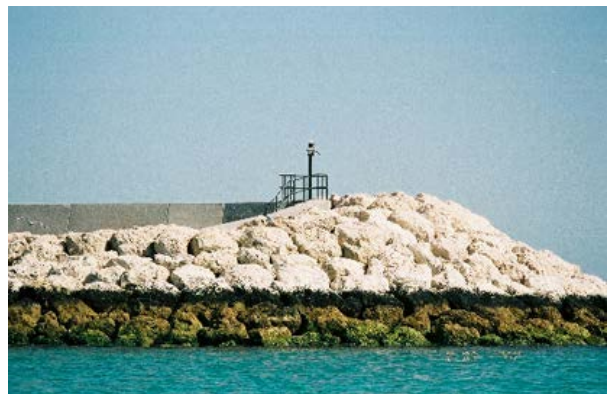
Mina Salman—Khalifa bin Salman jetty light
