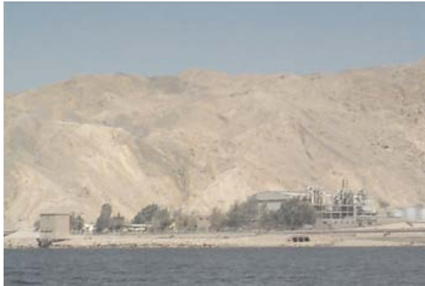
Al Aqabah—Power Station
