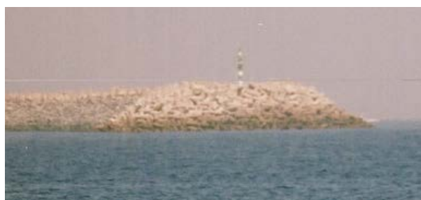
Fujayrah—South Breakwater Head
