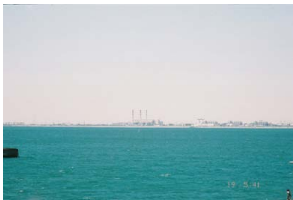
Aden Outer Harbor—Power plant chimney
