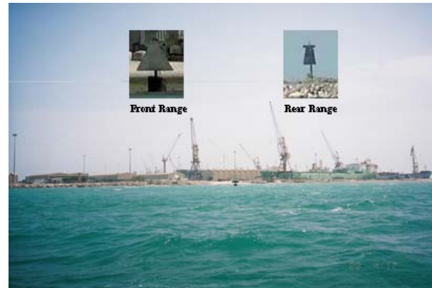
Deep Water Pier—106°54' outbound range
