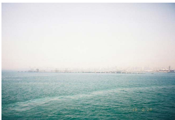
Mina Ash Shuaybah—Petroleum Products Pier from ENE
