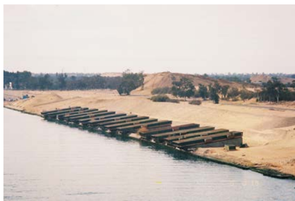
Pontoon bridge—Ready for deployment
