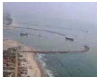
Karaikal Port Breakwaters
