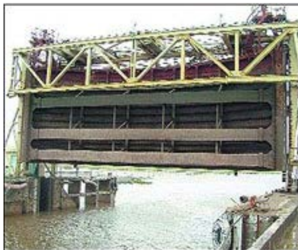
Lock Gate at Bhavnagar Port
