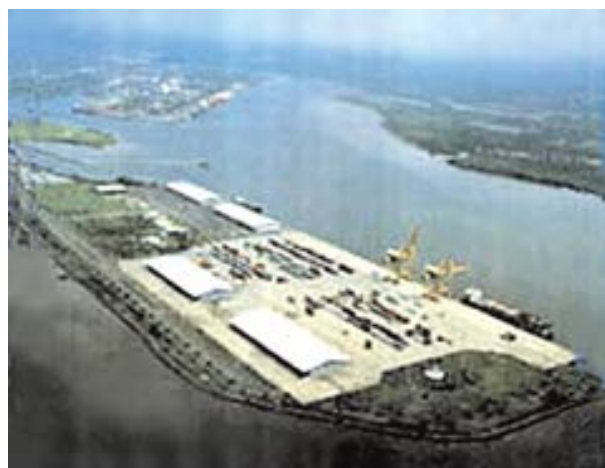
Belawan Container Terminal
