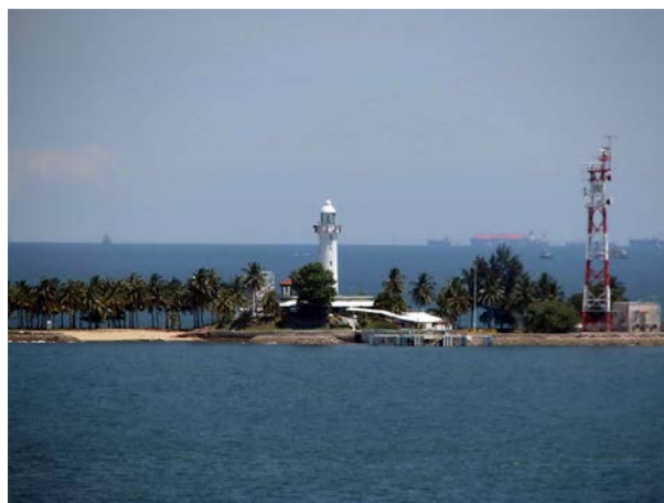
Raffles Lighthouse with VTS tower
