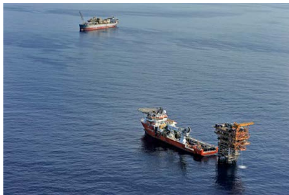
Montara Oil Terminal
