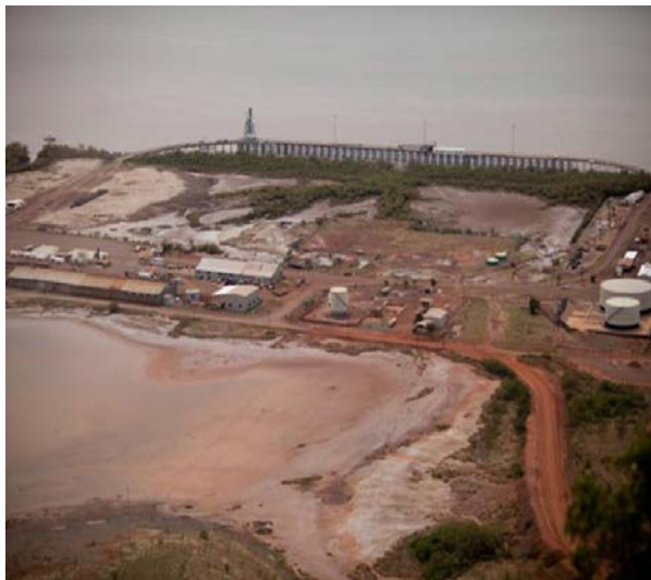
Wyndham Port Facility
