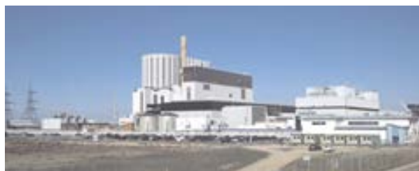
Dungeness Nuclear Power Station
