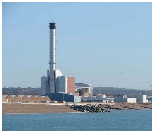
Shoreham Power Station
