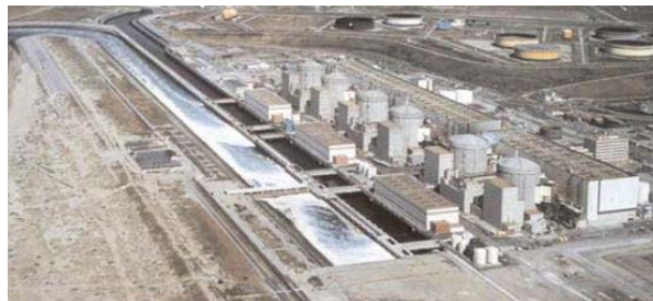
Gravelines Nuclear Power Station
