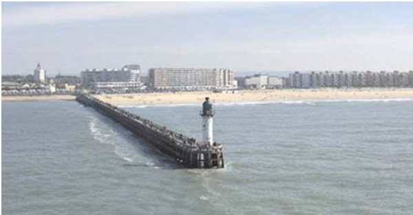
Calais West Jetty Light
