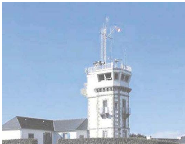
Ile de Brehat Signal Station
