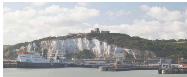
Ferry Terminal with Church Tower and Dover Castle on cliff
