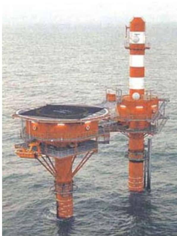
Oost Dyck Radar Tower
