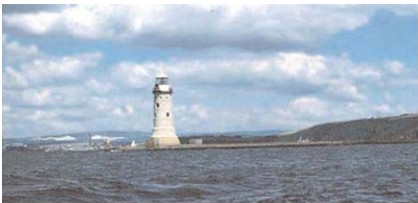
Plymouth Breakwater West Light
