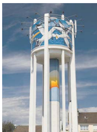
Calais—Bleriot-Plage water tower
