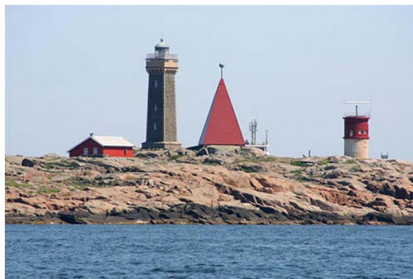
Vinga Light, day beacon, and radar tower
