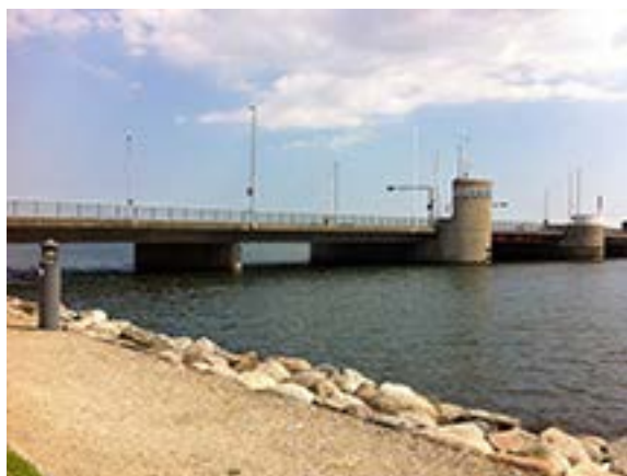
The Hadsund Bridge
